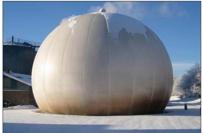
**Figure 3:** The gas buffer storage of 1000 m<sup>3</sup>
