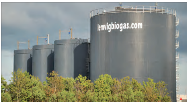
Figure 1: General view of Lemvig Biogas Plant (Photo: Lemvig Biogas)
