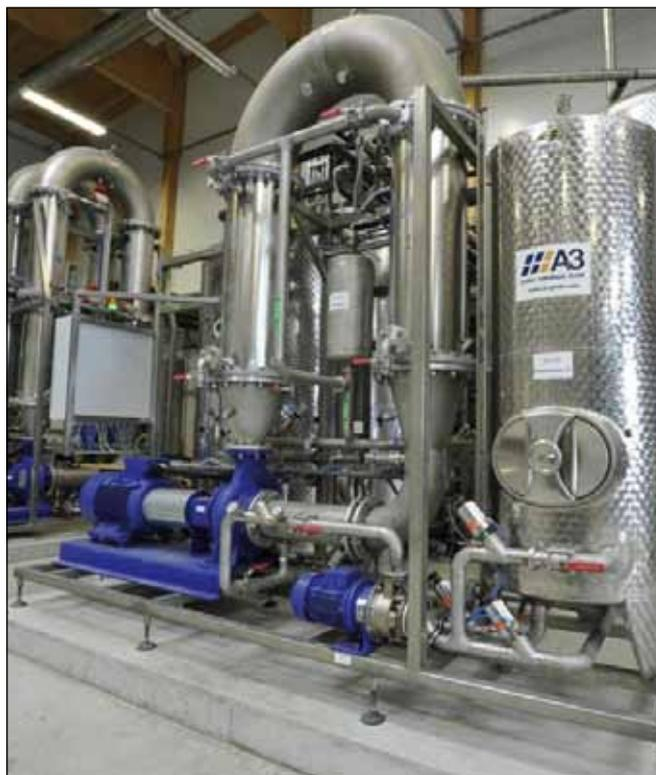
**Photo 2:** Ultrafiltration unit (Photo: SFPI)
