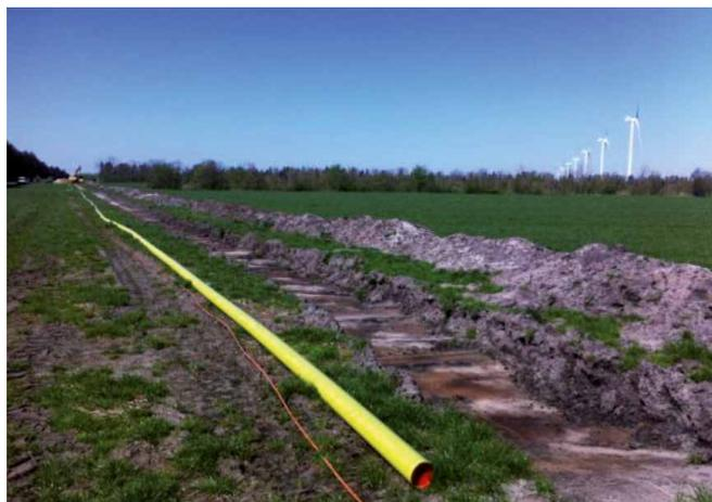
**Figure 4:** Biogas pipes being installed to connect biogas plants with local CHP units
