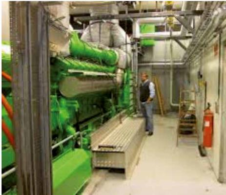
**Figure 6:** A 4MW gas engine for CHP-production
