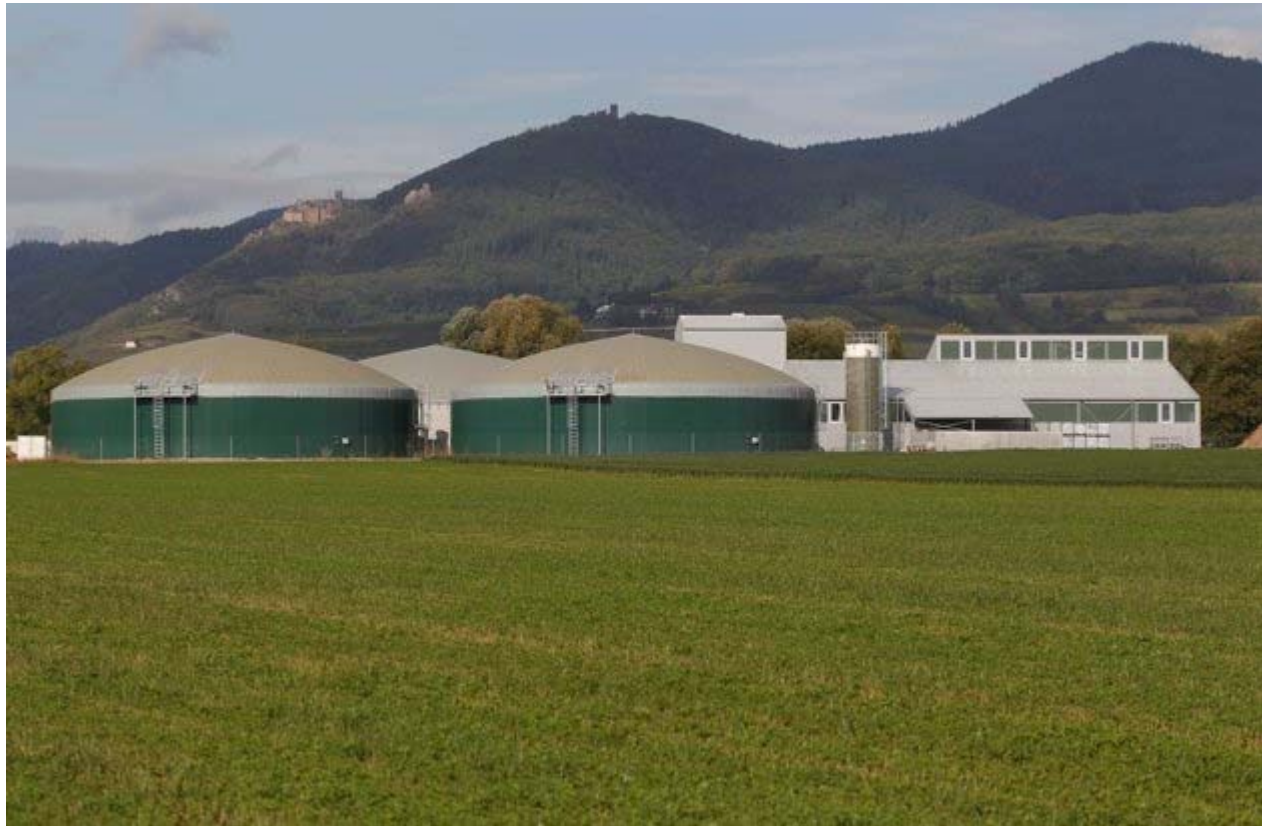
Centralised plant AGRIVALOR (Ribeauvillé, Lorraine) 26 000 tons capacity 1400 kWe and district heating system for a casino's swimming-pool
