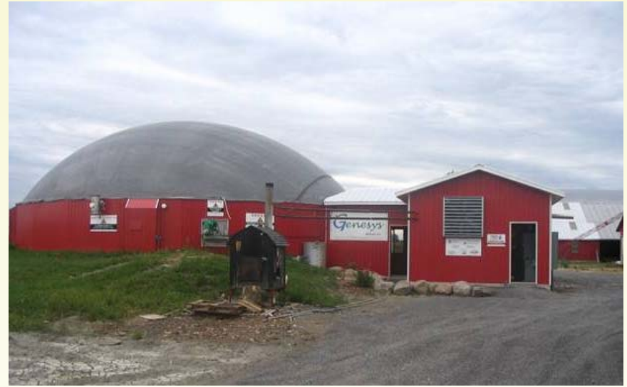
Terryland Farm Digester (St. Eugene, Ontario)
