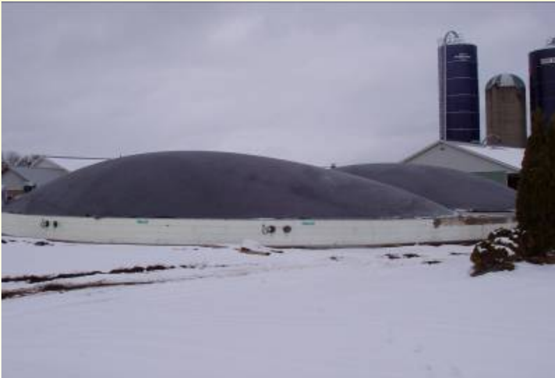
Fepro Farm Digester (Cobden, Ontario)
