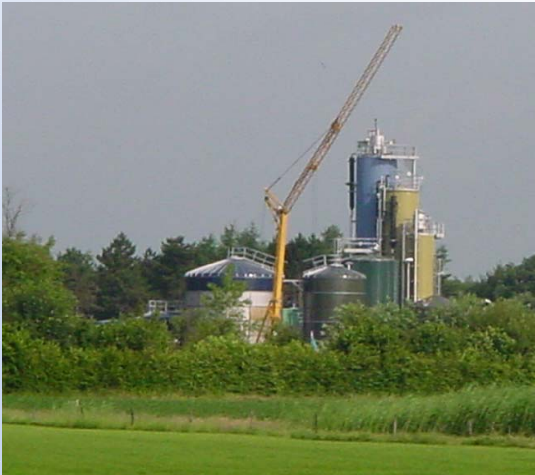
Construction of animal waste digester
