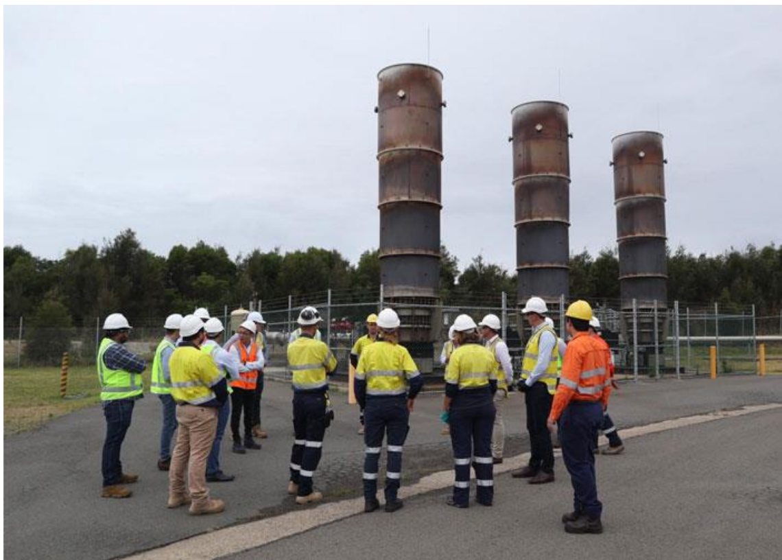
Figure 3.2. Flares on the Sydney Water Malabar Wastewater Treatment Plant that currently flare biogas
