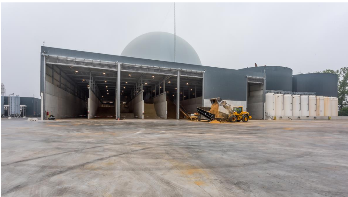
Figure 16.1. Aben BV biogas plant in Westdorpe
