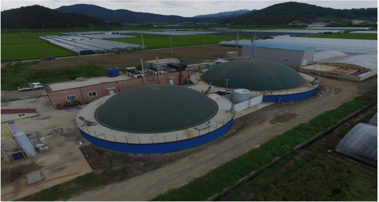
Figure 13.1. Chungyang Biogas Power Plant that is producing 8.16 GWh electricity (3,900,000 Nm 3 biogas) annually. Source: Chilsung Energy Farming Association, Chungnam, Korea
