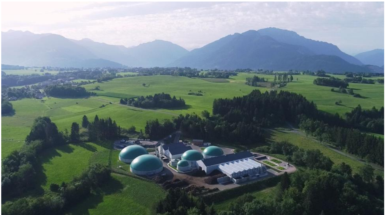
Figure 10.2. Collective unit in Vinzier, French Geneva Lake area, owned by Terragr'Eau Co (picture: GRDF). The plant uses various products from agro food biowaste and manure. This is the first French plant that uses an amine scrubber to clean the biogas.
