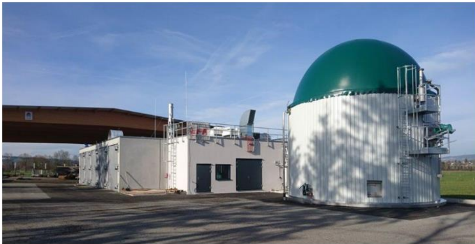
Figure 15.2. Expansion of an existing composting facility (rear) by Dry AD (centre)
