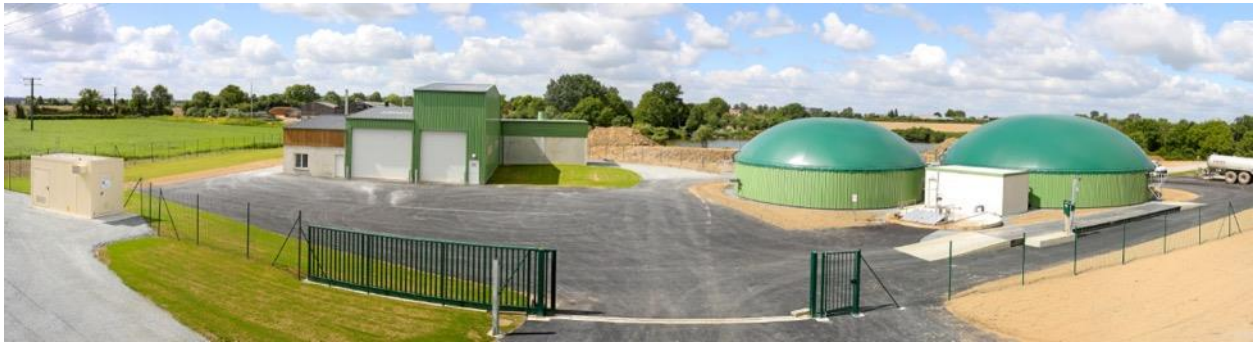
Figure 10.1. Collective unit in Mortagne sur Sèvre, west of France, owned by Agribiométhane Ltd. (picture: GRDF). The plant produces biomethane from manure and agri-food wastes. This is the first French plant that uses a PSA system to clean the biogas.
