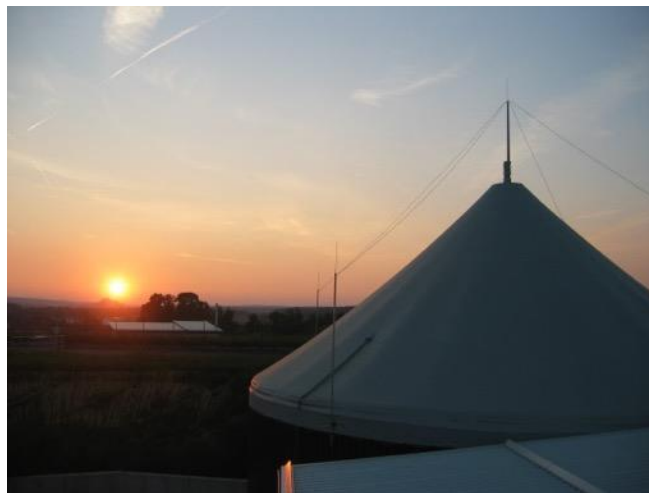
Figure 4.1. Biogas plant in Strem nearby Güssing
