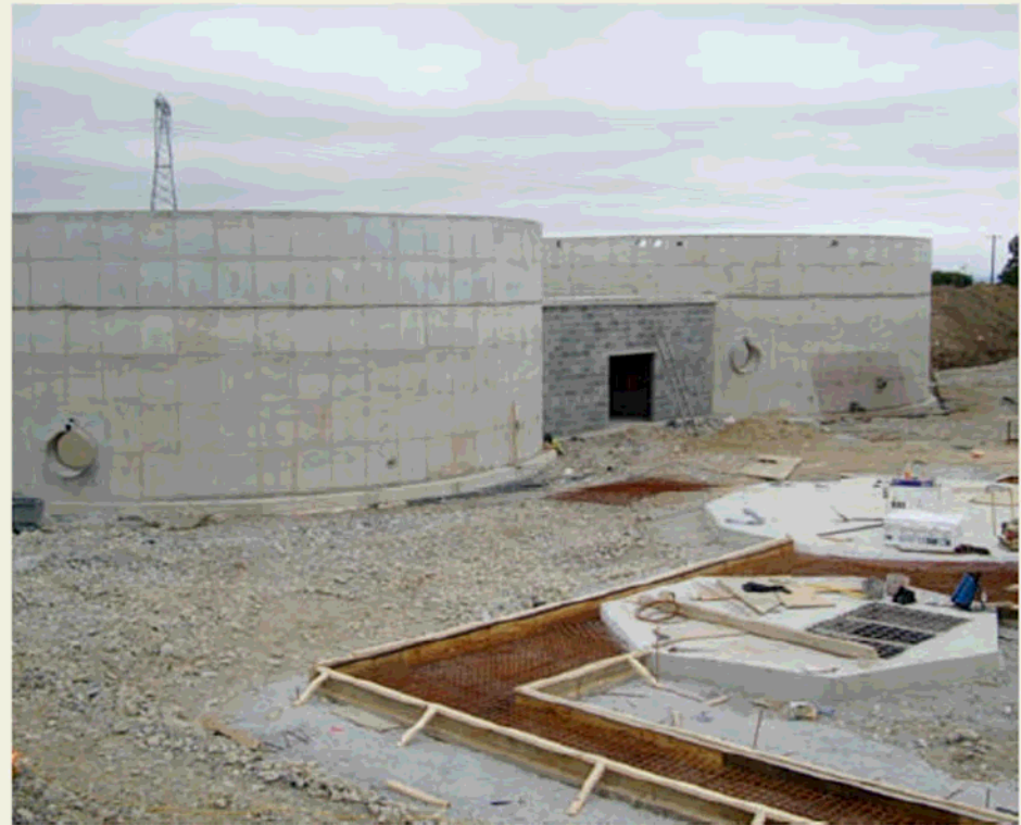
Completed tanks and reception building preparation.
