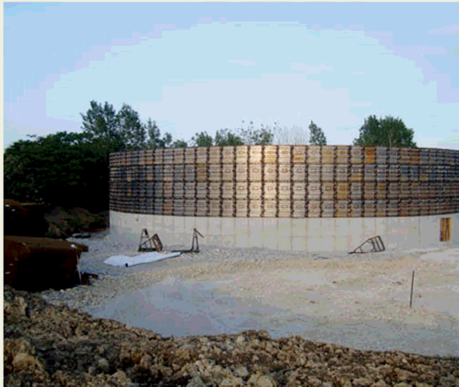
Completed tank wall.
