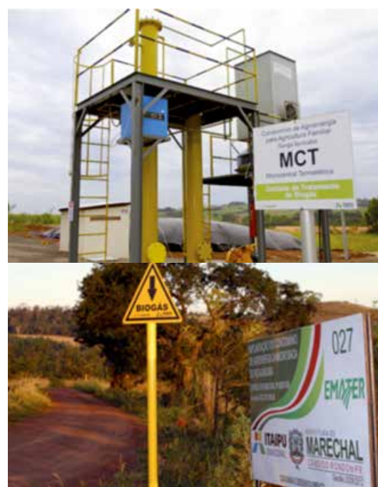
Figure 10 Small biomethane upgrading plant in Brazil; top: pilot biomethane upgrading plant which serves a co-operative of 33 family farms with an aggregate of 100 LSU, Capital cost: £66,000, Biogas throughput: 5 Nm 3 /hour (Photo: ITAPU Binacional, Brazil, 2014); bottom: biogas is transported through a pipeline to link the farms to a central CHP adjacent to the new upgrading plant.(Photo: Clare Luke-hurst)
