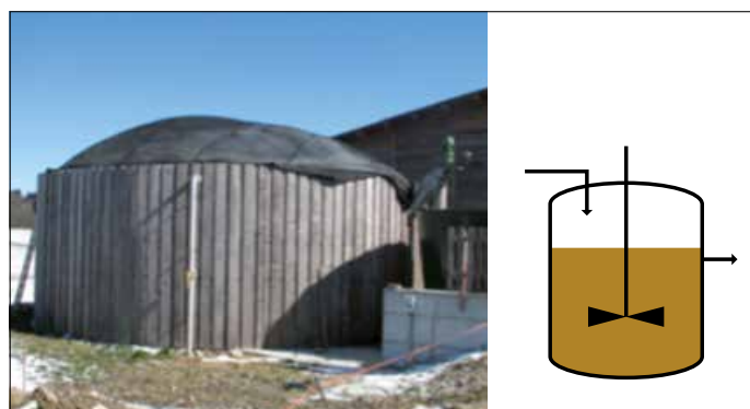
Figure 4 'CSTR' digestion system at Saugealles Fermes, Switzerland (Photo: EREP SA)
