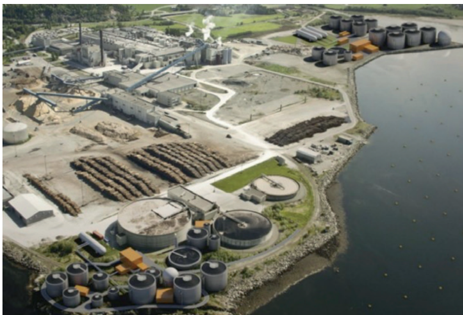
Figure 3. Biokraft biogas plant in Trønderlag in Norway is positioned at the harbor and close to Skogn pulp and paper plant. The plant uses residual products from the pulp and paper industry and the fish farm industry as substrates and has the capacity to produce about 25 million m 3 liquid methane for vehicle fuel per year.
