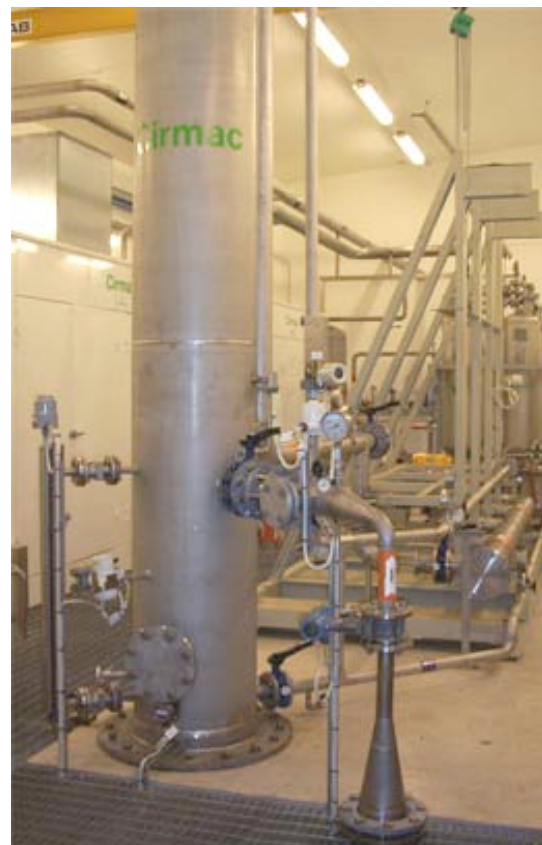
Chemical absorption plant, capacity 300 m 3 /h Borås, Sweden
