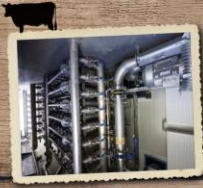
Gas to grid. We can inject 7 million m 3 of green gas to the grid every year – saving up to 15 million kgs of CO 2 per year.
