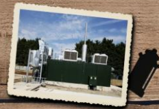
Sustainable cheesemaking. CHP machines, using the biogas from our AD plant, generate over 8 million kwh of electric – saving over 5 million kgs of CO 2 per year.
