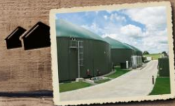
AD plant. Generates biogas using farm and dairy waste.
