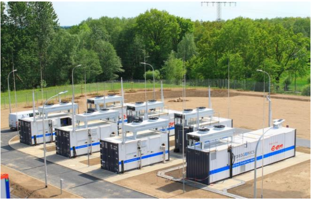
2 MW Power-to-Gas unit (Falkenhagen, Germany). Hydrogen is injected into the grid without methanation
