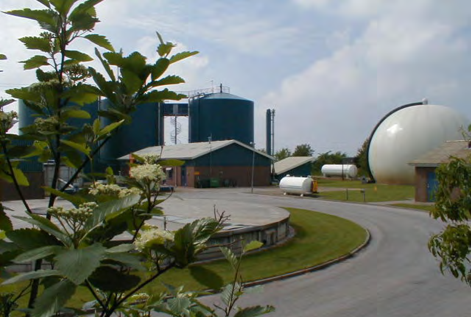
Ribe Biogas; 15 years of production, 18.000 m 3 biogas/day. Source J. B. Holm-Nielsen, Bioenergy Dept., SDU, Denmark.
