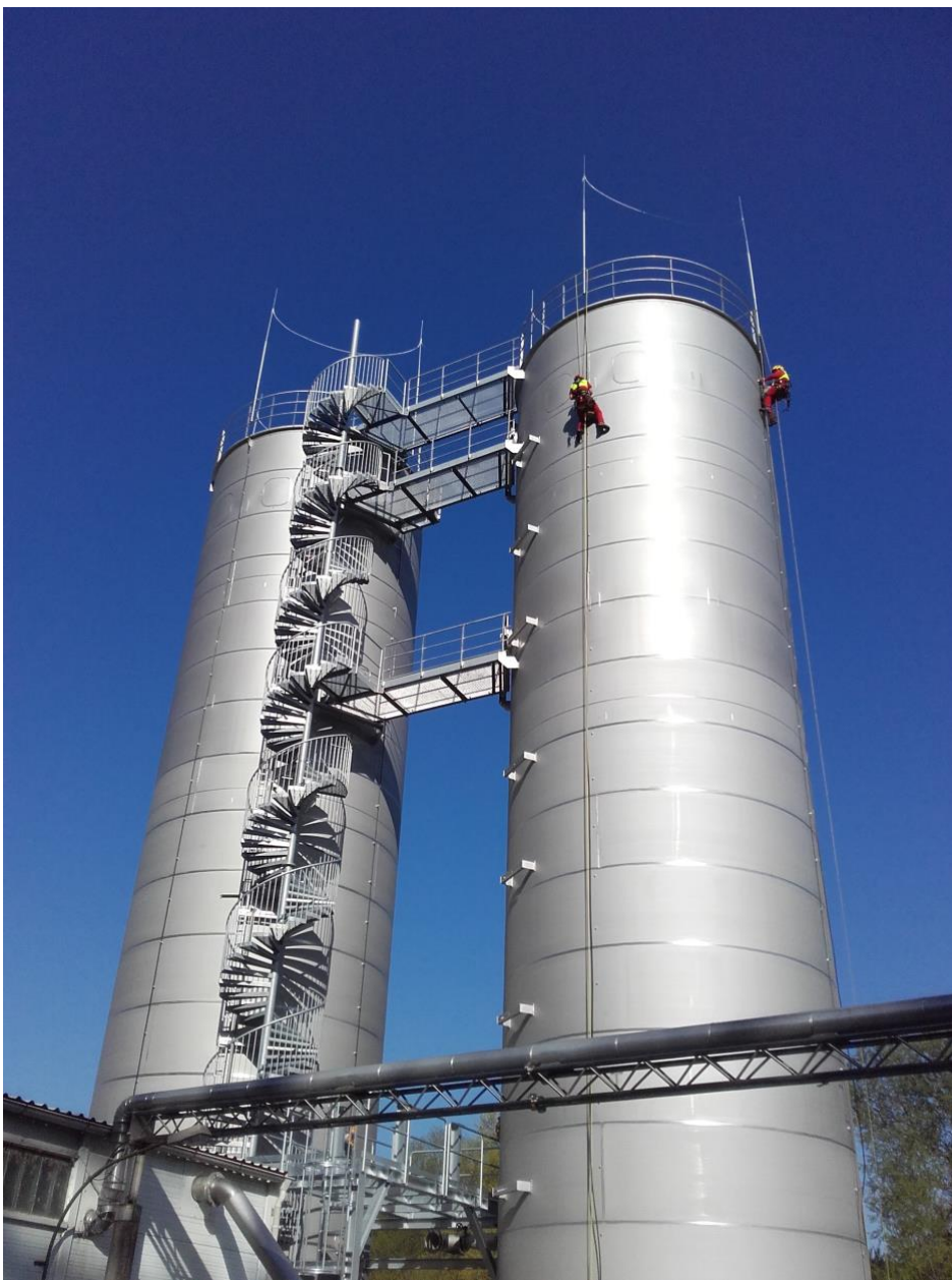
Figure 3: IR-Reactors at the wastewater treatment facility.
