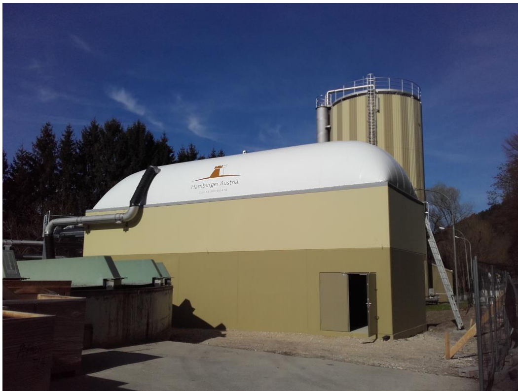
Figure 2: Wastewater treatment facility at W.Hamburger facility in Pitten,
