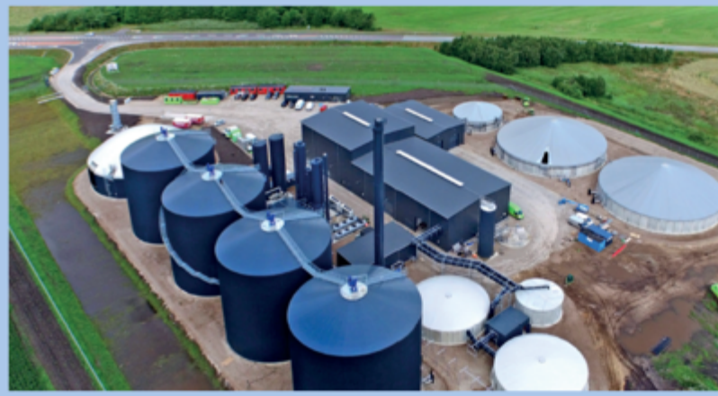
Figure 3: Holsted Biogas Plant, producing 20.7 million m 3 gas / year. Source: Nature Energy
