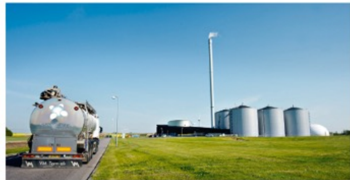
Figure 1: General view of Maabjerg BioEnergy Plant, (Photo: Maabjerg BioEnergy)
