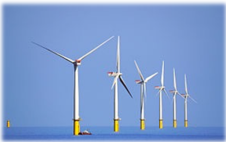
Walney wind farm extension, built in 2017, has a 659MW capacity and cost €1.4 billion.
