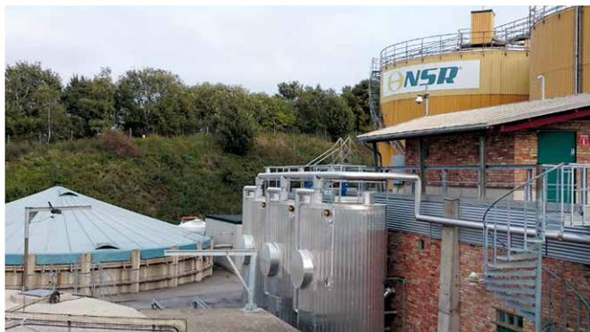
**Figure 4:** To the left, the digestate storage tank from which the digestate is transported to farmers by pipe-line or truck. To the right the heating tanks for the hygienisation process.
