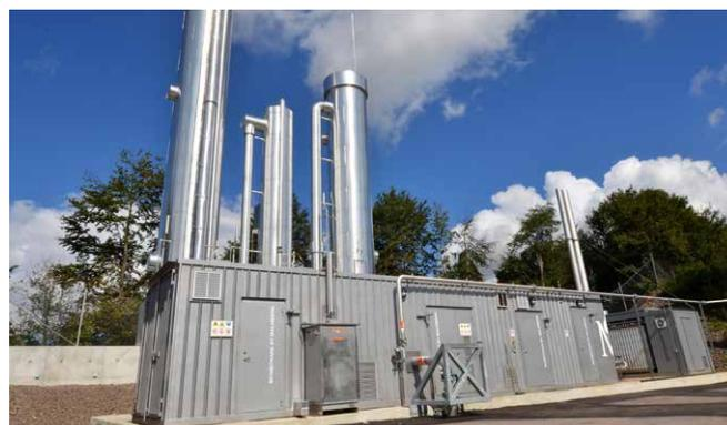
**Figure 5:** The biogas upgrading plant based on water scrubbing technology with a capacity of 1400 Nm<sup>3</sup> raw biogas/h.
