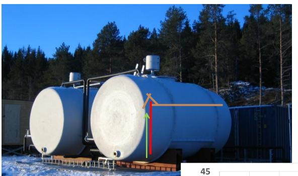
Due to loss of culture the plant experienced low biogas yield. A barrier was introduced (January) to improve retention (see left). => increased biogas yield (below) (Low production in mid Feb caused by unitentional blocking by ball of straw)
