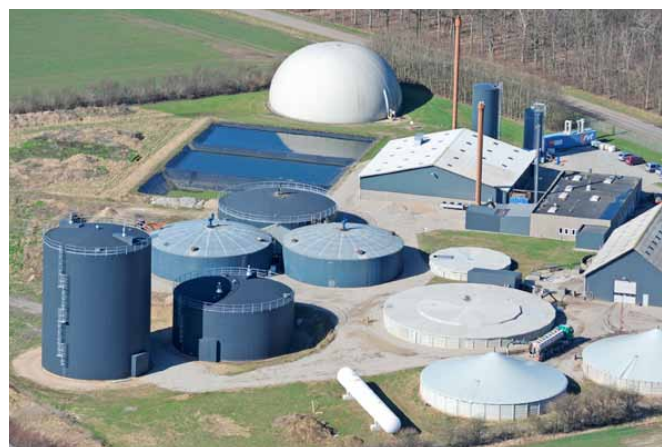
Figure 1: General view of the Linko Gas Biogas Plant (Photo: Linko Gas)
