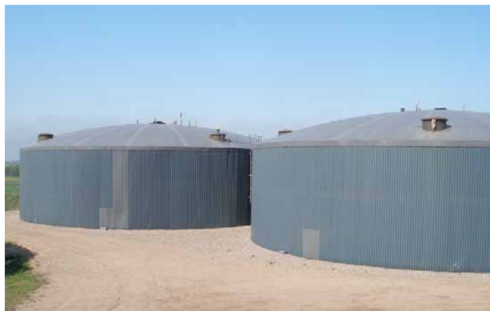
Figure 2: The digesters of 2400 m 3 each. (Photo: Linko Gas)
