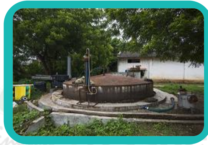
Community based Biogas Plant (25-1000 m 3 )
