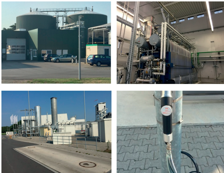
Figure 4.1: Audi E-gas power to methane facility at Werlte, Germany; From clockwise top left: food waste digester; 6 MW alkaline electrolyser; hydrogen service station; overarching view of catalytic power to methane system
