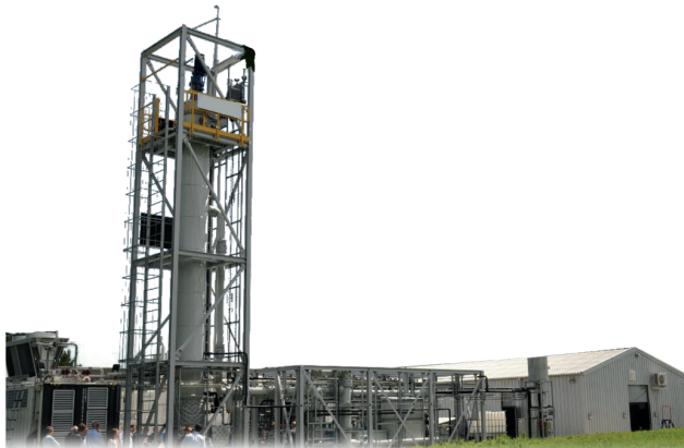
Figure 4.3. Photograph of BioCat Plant on BIOFOS site in Avedøre (from Power-to-Gas via Biological Catalysis (P2G-Biocat))
