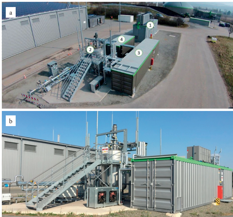
1. Proton Exchange Membrane electrolyser. 2. Methanation reactor 3. Measuring and mechanical process 4. Process and control
