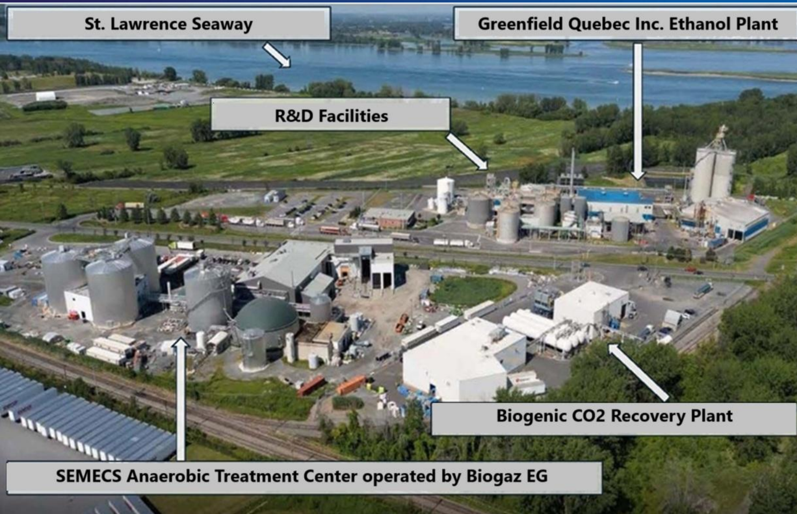
Greenfield Global Biorefinery Complex in Varennes, Québec (Canada)
