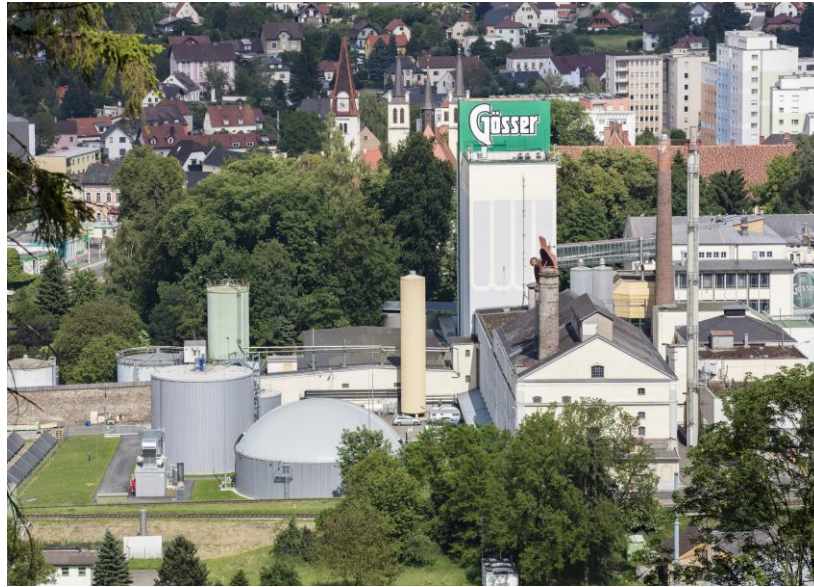
Figure 12 Biogas plant at Gösseer Brewery in Leoben, Austria (reproduced with the kind permission of BDI-BioEnergy International GmbH)
