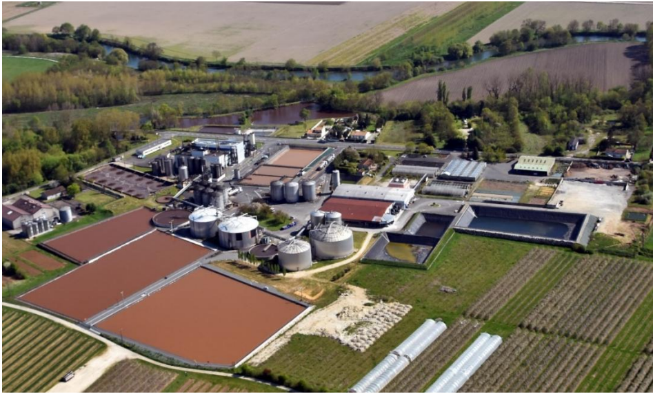
Figure 16 Biogas plant in St. Laurent de Cognac, France (reproduced with the kind permission of REVICO)
