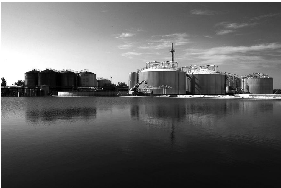
Figure 15 Biogas plant in St. Laurent de Cognac, France (reproduced with the kind permission of REVICO)
