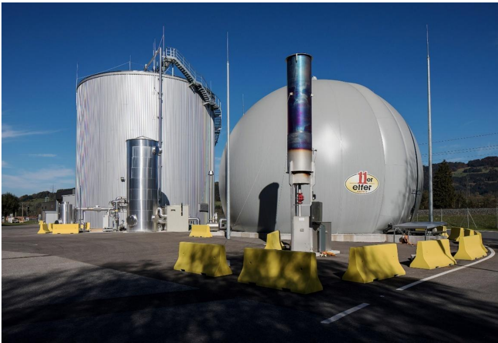
Figure 17 Biogas plant treating potato processing by-products in Frastanz, Austria (reproduced with the kind permission of 11er Nahrungsmittel GmbH)
