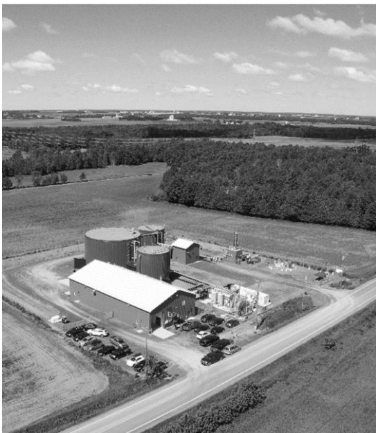
Figure 1: Coop Agri-Energie Warwick AD facility (Coop Agri-Energie Warwick, 2024)
