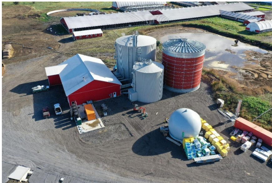
Figure 2: GET Corp. Pilot AD Project in Brinston, Ontario (GET Corp., 2024)
